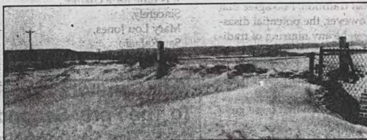
Drifting sand along NM 605 North buries a fence line.
