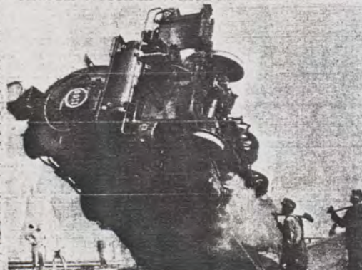
One of the largest locomotives in use on the Pennsylvania Railroad system was left in this precarious position after its train split a switch on Ohio Crossing bridge near McKees Rocks. Rear of engine broke through the span
